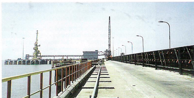
Fig. 4: Straight portion of pipe conveyor at jetty
