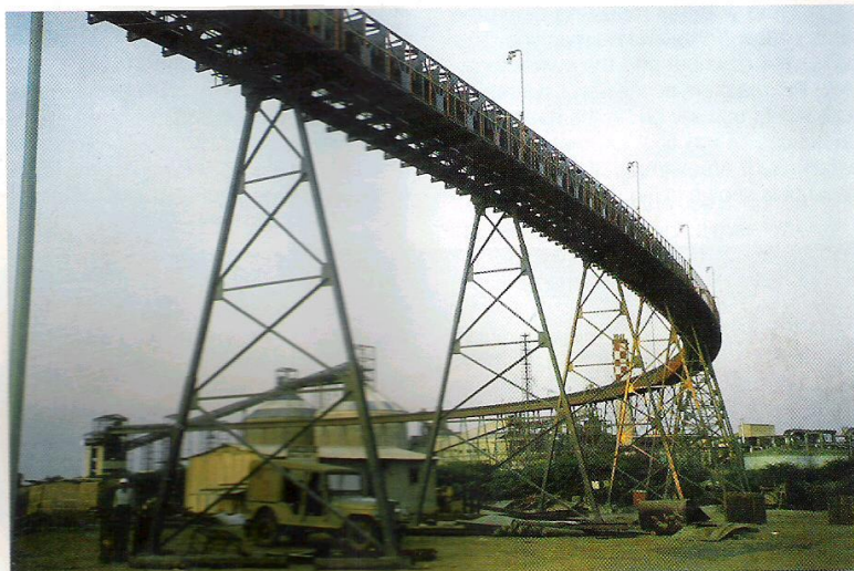
Fig. 1: 3.2 km long pipe conveyor at Birla Copper
